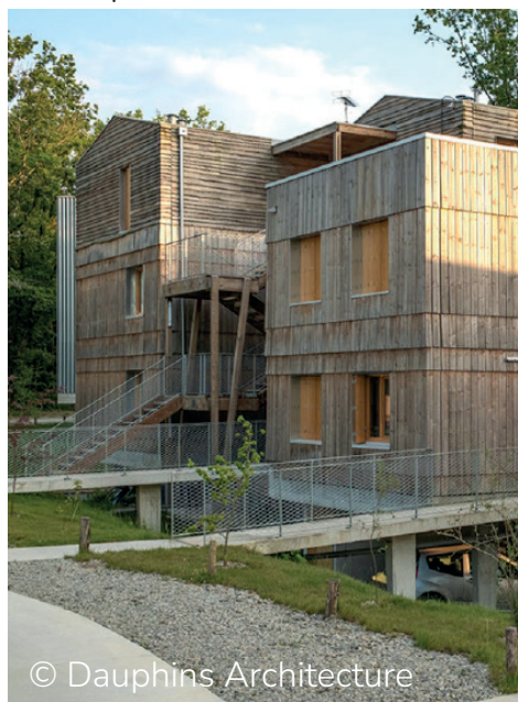
Mouline Sud, Ambarès (33) - Dauphins Architecture
